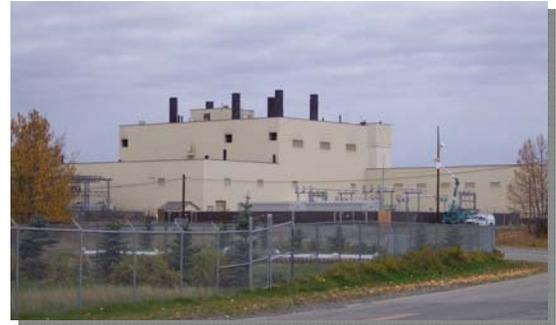
This challenging project scope was completed in two short Alaska construction seasons. The decentralized boilers were commissioned and running and the CHPP was shut-down on schedule for the start of the critical heating season.
