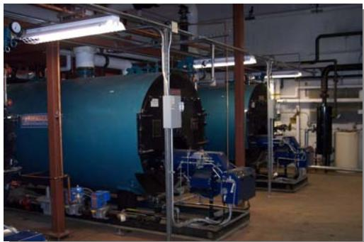
Each boiler plant is sized to serve the building in which it is located. In order to provide freeze protection against boiler failure, each building has at least two steam boilers, each sized for 60% of the peak building load.
