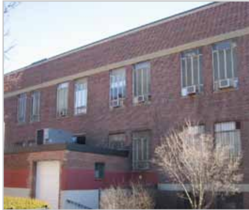
The window units will be replaced at the Authority's administrative building.
