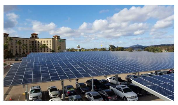
A 936 KW solar carport array installed on a Federal Aviation Administration compound in California through a performance contract with a local utility company. Photo by Joe Garrido.
