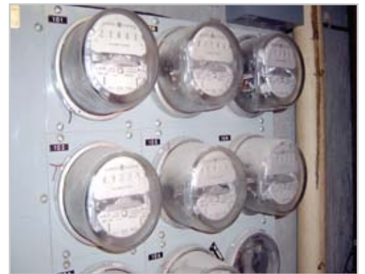
Work is already under way to improve the heating system, which will lower energy use and result in cash savings and a more comfortable living environment.
