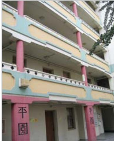
Ping Yuen will feature a new heating system and energy-efficient lighting.
