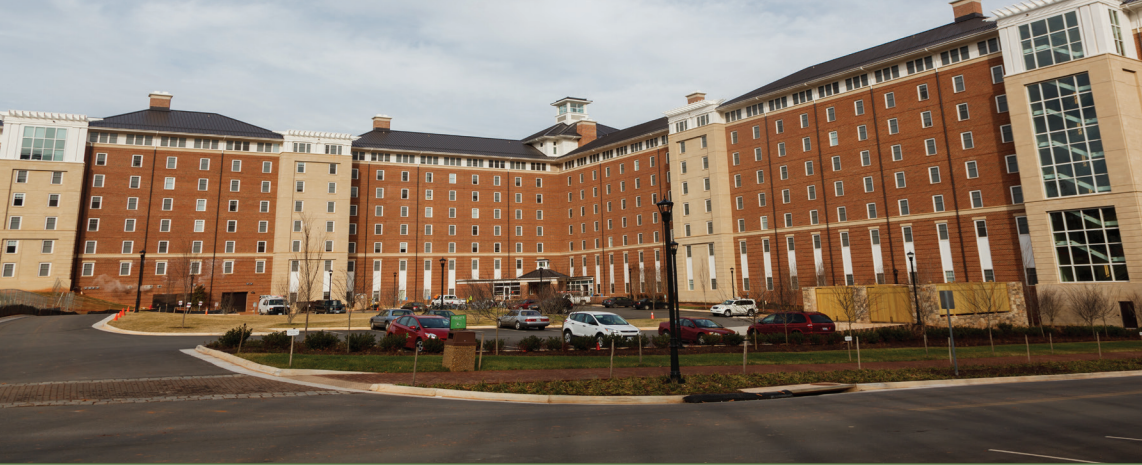
Wireless, energy-saving occupancy sensors in each residence hall room helped meet aggressive construction time lines.
