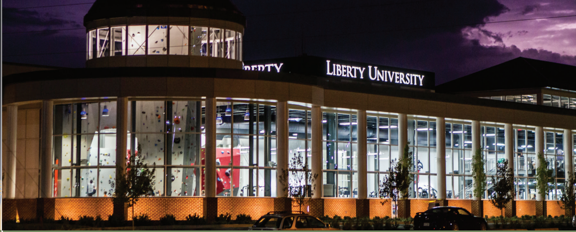
Liberty's expansion plans include lighting control systems throughout campus buildings, such as the LaHaye Student Union (shown above)
