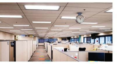
maximum flexibility, the project team created 3,685 control-integrated fixtures, installing McWong's TruBlu low voltage passive infrared occupancy sensor controller in each fixture and connecting it via a 0-10V output with the LED driver. This enabled the new fixtures to directly replace existing fixtures without the need for any additional wiring, a significant savings in labor and materials costs. In addition, the same fixture-level control was added to 225 existing fixtures.
