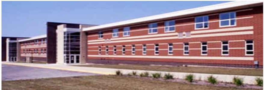
CTS Group designed renovations at McHenry West High School, installing an energy efficient HVAC system, geothermal loop system, and building automation system, saving over $255,000 annually.
